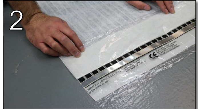
2 Lay back the white flaps on the long sides of the mats to expose the clear film with metal conductor bars and black heating elements.
