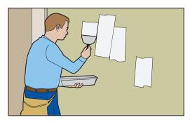
• Make repairs and remove any loose paint, wallpaper and all other contaminates that may affect adhesive bond (prime & paint repaired areas).
