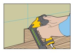
Use a level to double-check the levelness of the line between the two marks. Adjust line as needed with spacers. Secure this first row fully using adhesive and 2' finish nails or wood screws into pre-marked wall studs, placed approximately 2" above subfloor (these will be covered by your baseboard trim).
